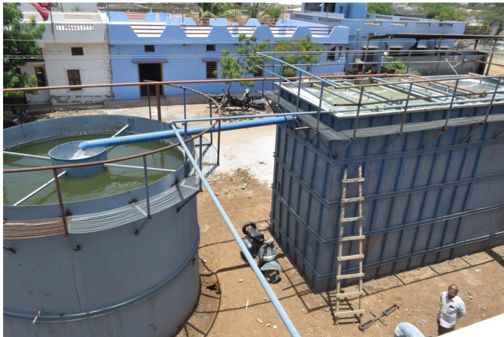
Fig.2: Secondary Clarifier and MBBR cum Aeration Tank
