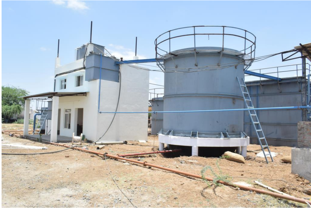
Fig.1: Reaction Tank & Settler-1
